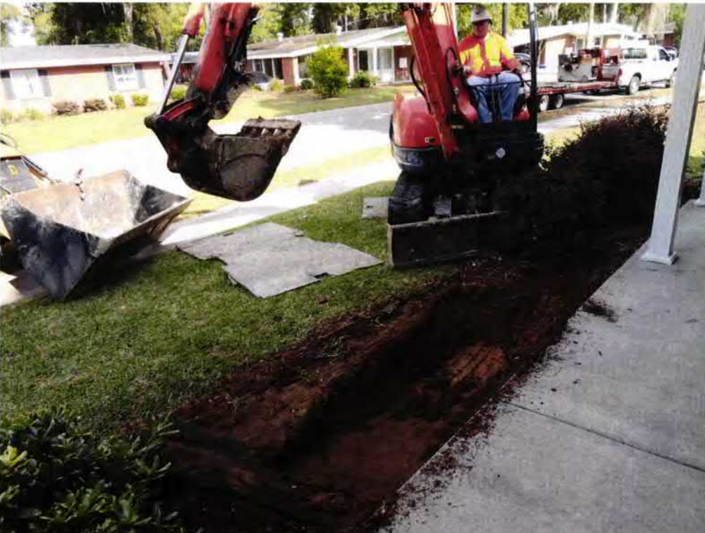
Picture 2: UST 603Dahlia excavation in progress.
